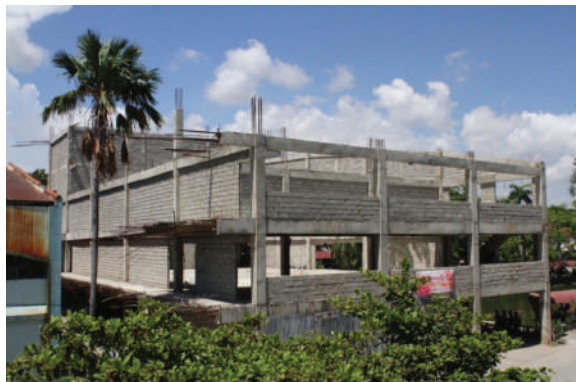
Front View of the On-Going UNP Gym
